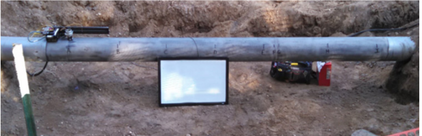
Pipeline Integrity Assessment
